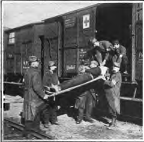
A FRENCH HOSPITAL TRAIN OF FREIGHT CARS, WITH STRETCHERS SUSPENDED TO ABSORB SHOCKS
